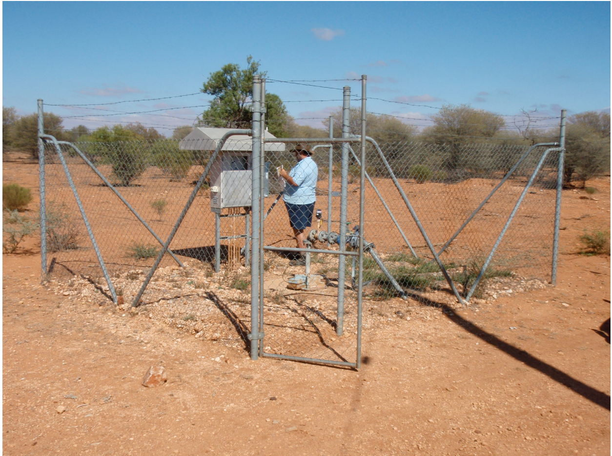
Photograph 2: Bore 2 – potable supply bore
