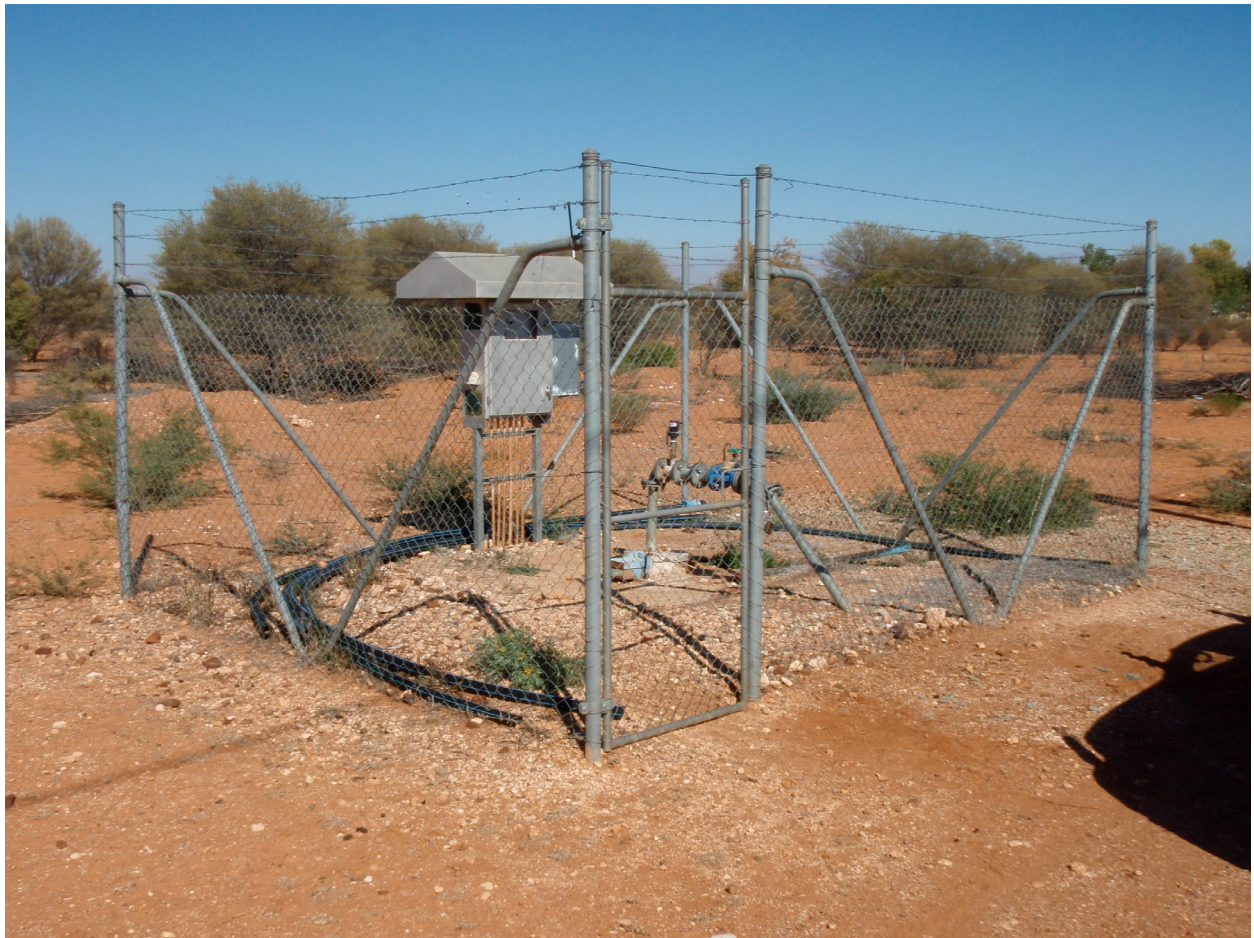
Photograph 1: Bore 1 – potable supply bore
